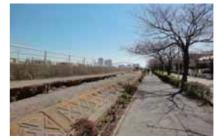
Bumped seawall caused by liquefaction Photo: Chuo Kaihatsu
