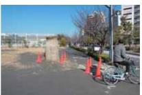
Uplifted manhole by liquefaction Photo: Nihon Suido Cosultants
